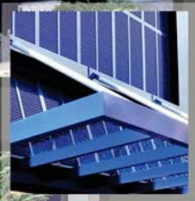
Metal Canopy with Glass Roof
