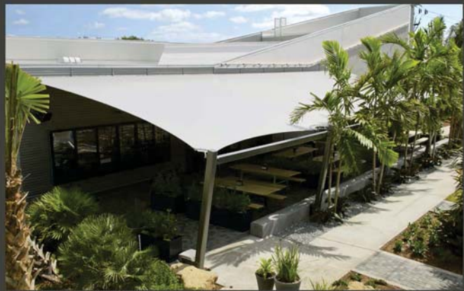
Tension Structure over Outdoor Dining Area
